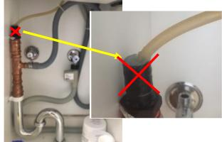
Note these tundishes have been sealed, preventing the drain pump from pumping against back pressure. This also results in phantom alarms as the machine senses pressure back from the waste system into the tub level pressure sensor
